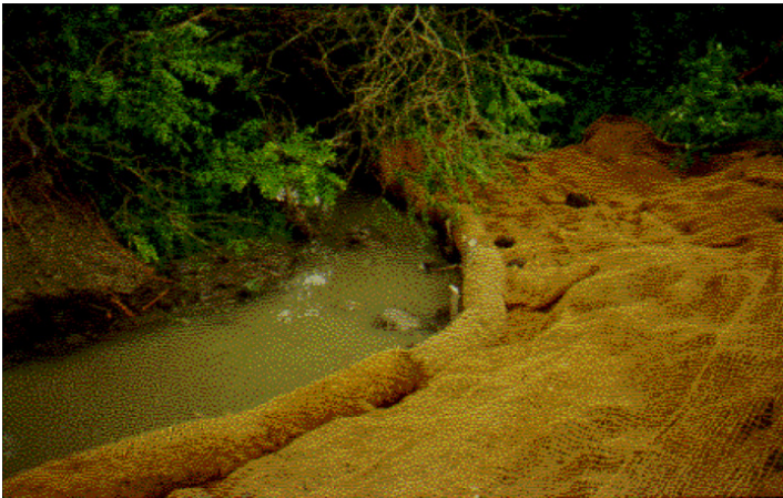
Figure 11: application of the coconut fiber rolls in a wet ground, (IDNR, 2006)
