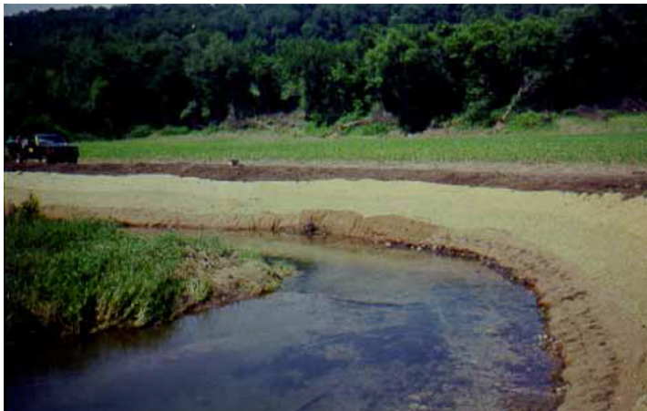
Figure 8: Streambed which has been graded and seeded (IDNR, 2006)
