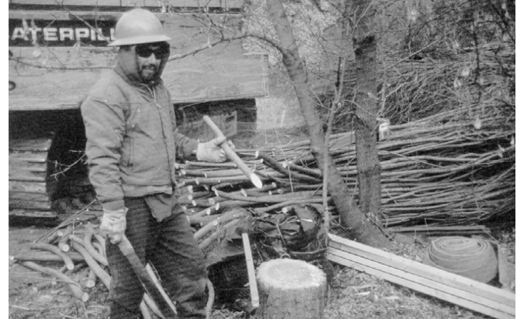
Figure 9: preparation of the live stakes, (IDNR, 2006)
